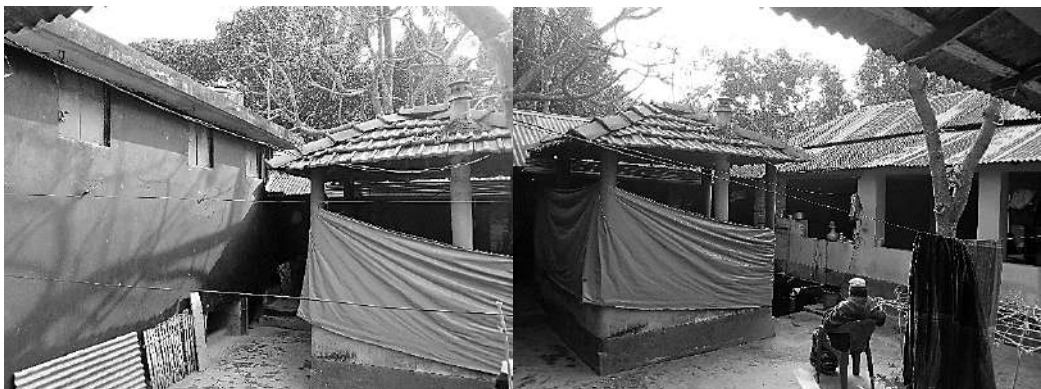
Figure: Transformed Gola Ghor with modern materials and non-transformed kitchen's roof materials (Photograph by author)
