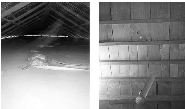
Figure: Showing the TALA space where some paddy is keep for drying and second image showing the below part or TALA. (Photograph by author)
