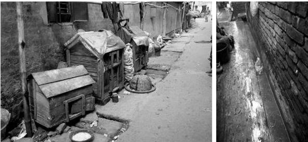
Figure 10: Covered drain and open drain used as waste water discharge of the Rupsha char community (Source: Author, MSCHS Studio 2017)
